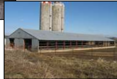
48x27 Grade A Milk Barn 7/Side; 14 Orbit Milking Heads
